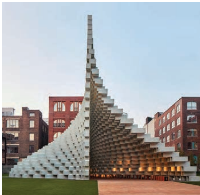
The Serpentine Pavilion at KING Toronto Bjarke Ingels
